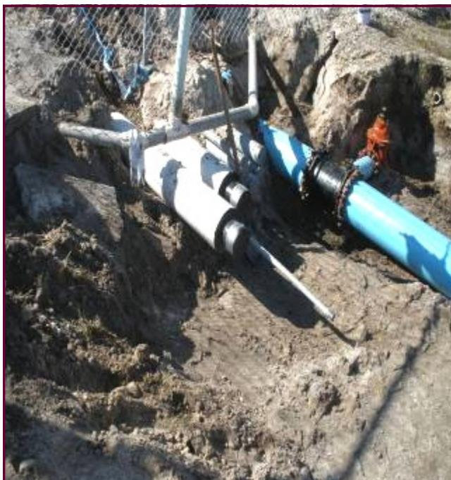
A water line has been constructed onto the District property. This water line is a requirement both by the Health Department and the Fire District prior to new construction of buildings at Buckingham. This was the first phase to the new Administrative Building. This project required a 600 foot directional bore under the taxiway.
